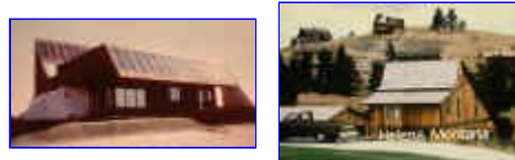
solar integrated south facing roofs
